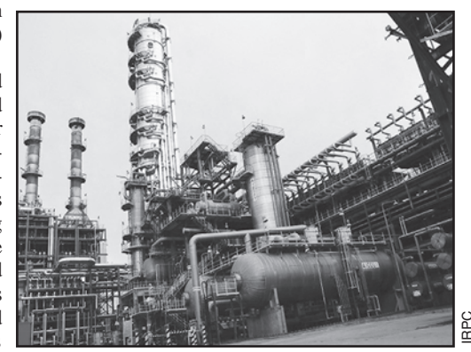
IRPC's Condensate Splitter at its Rayong province petrochemical complex.
