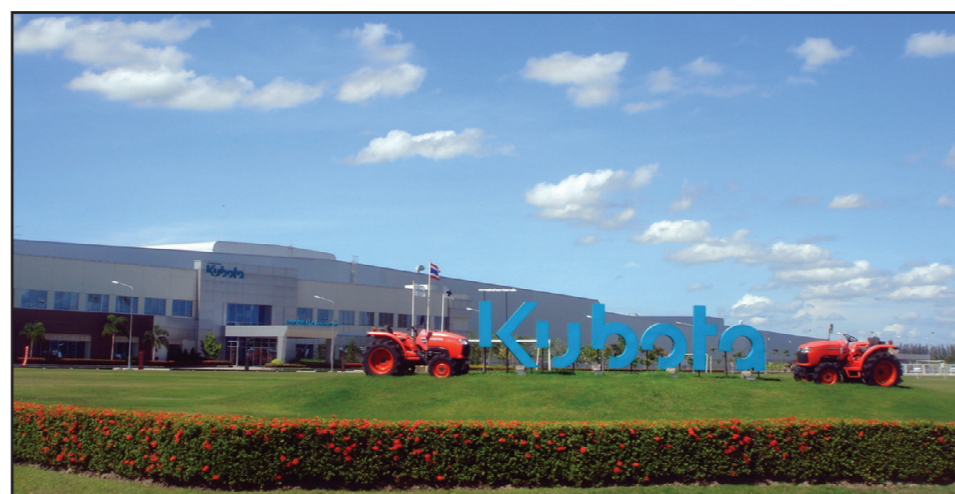
Siam Kubota's Amata Nakorn Plant in Thailand
