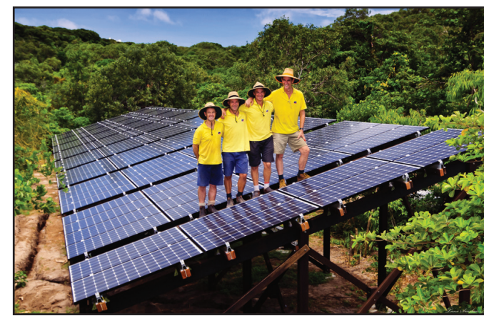
Panasonic solar installation at Lizard Island on the Great Barrier Reef, Australia
