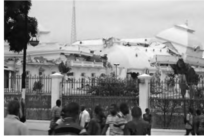
Symbol: The Haiti National Palace stands severely damaged on Jan. 12, 2010, in Port-au-Prince after a devastating earthquake struck. LISANDRO SUERO / GETTY IMAGES
