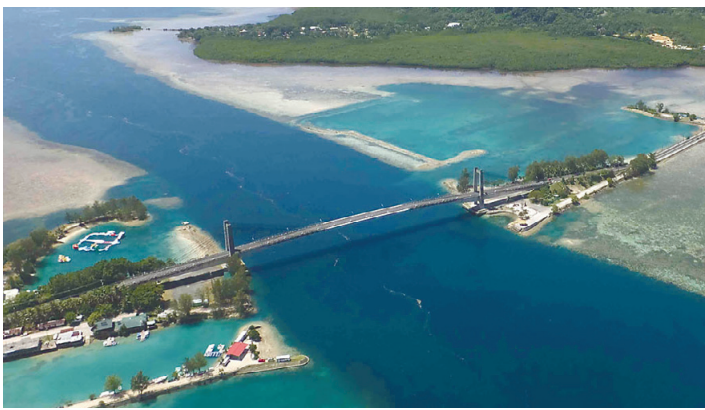
Clockwise from above left: Palau's famous Rock Islands; Enjoy the ultimate island style in Palau; K-B Bridge, or the Japan Palau Friendship Bridge, connects Koror and Babeldaob Islands. It is a reinforced concrete, cable-stayed bridge with a total length of 413 m. NARIHIRO TANAKA / EMBASSY OF PALAU
