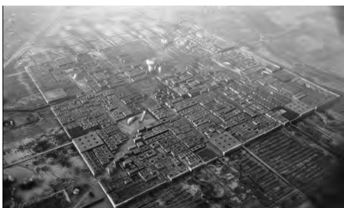
Masdar City: The world's first carbon-neutral, zero-waste city in Abu Dhabi serves as a new global hub for the intellectual and technological development of renewable energy.
