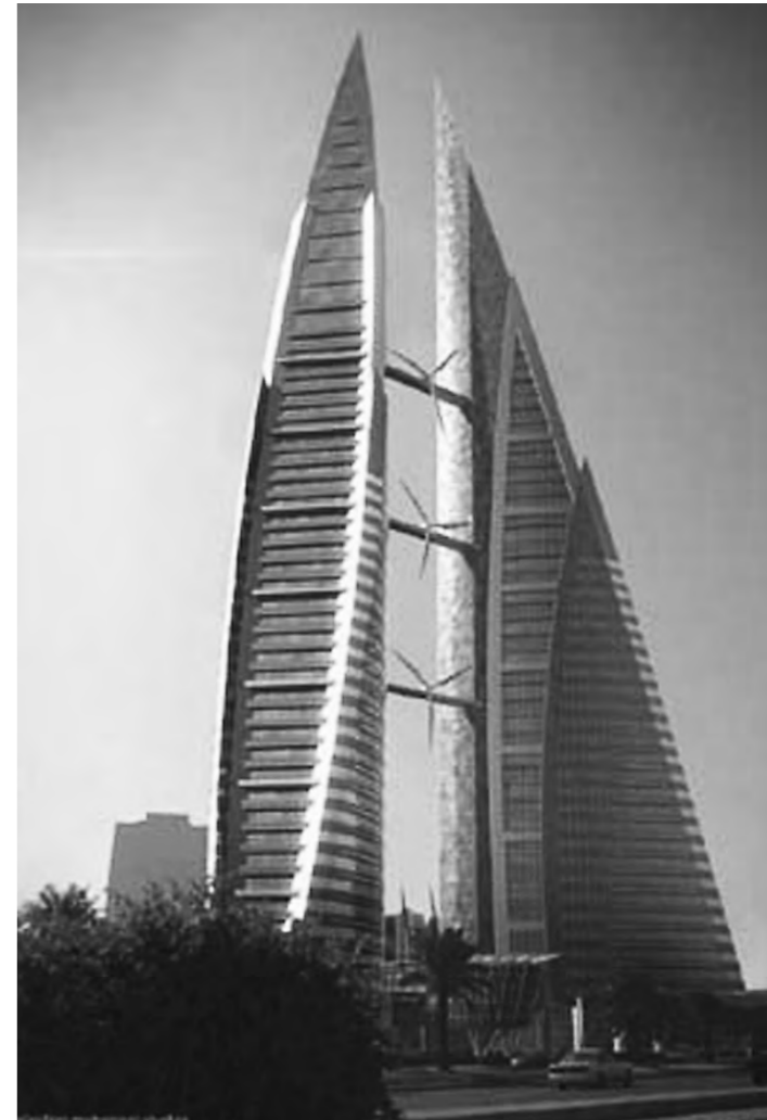
Open for business: Bahrain's World Trade Center is home to office towers, shopping malls and a five-star hotel, making it the ideal business location.
