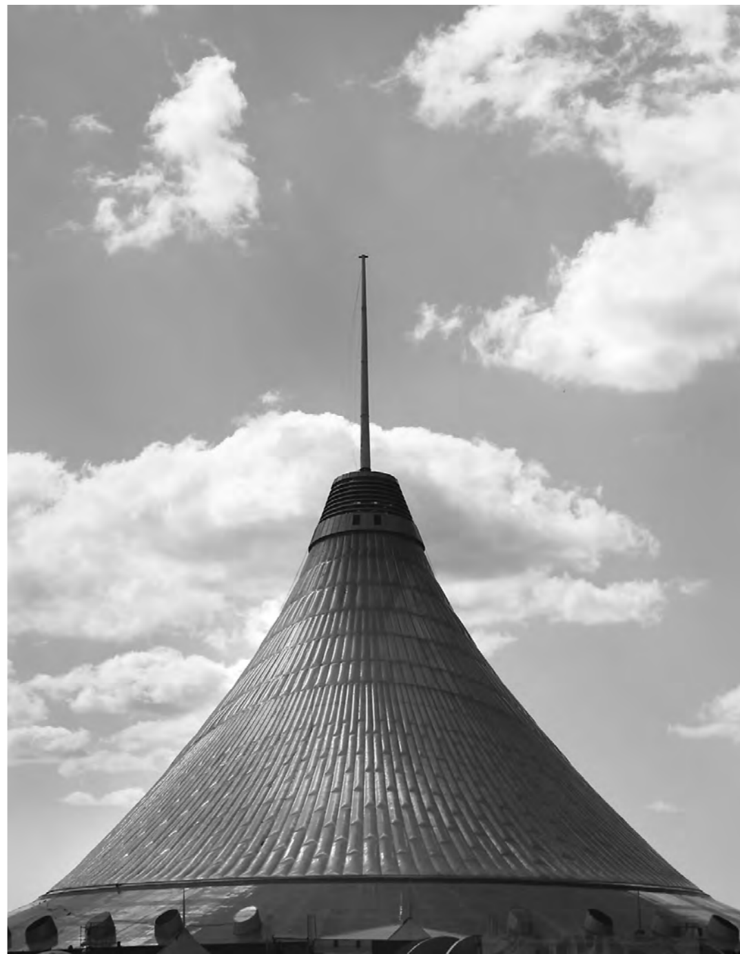
Futuristic: The Khan Shatyr Entertainment Center, designed by British architect Norman Foster and opened this July in Astana, has a 150-meter-high transparent tent over an area of 140,000 sq. meters — larger than 10 football stadiums.
