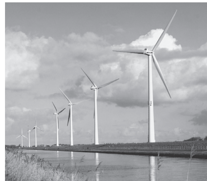
Clean energy: Modern windmills dot the Dutch coast to produce electricity. EMBASSY OF THE KINGDOM OF THE NETHERLANDS
