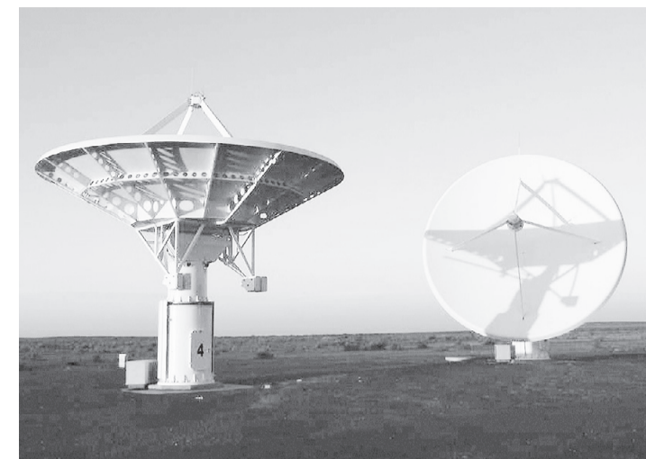
High-tech: The seven-dish MeerKAT precursor array KAT-7 in South Africa is the world's first radio telescope array consisting of composite antenna structures. EMBASSY OF SOUTH AFRICA
