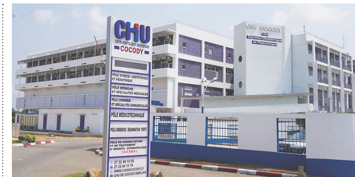
The Gyneco-Obstetric and Pediatric Unit of the Cocody University Hospital was built with a donation from the Japanese government.
