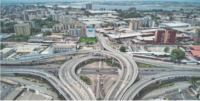
The Cocody interchange is a symbol of development in Abidjan. EMBASSY OF COTE D'IVOIRE
