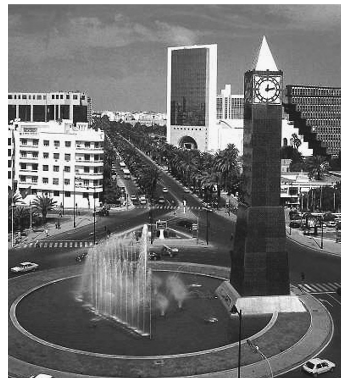
High time: A burnished metal clock tower provides a glimmering landmark toward the western end of Tunis' main thoroughfare.
