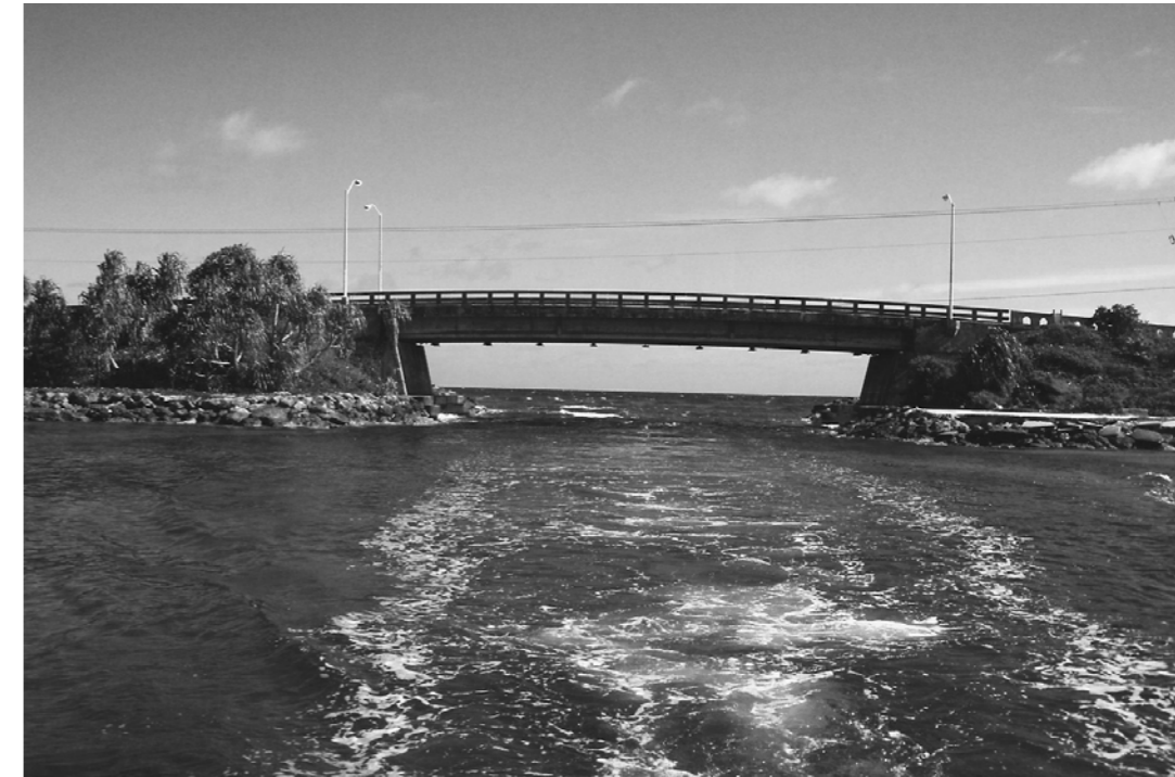
Bilateral link: Majuro Bridge (called Nakasone Bridge), the highest point in Majuro, was built with Japan ODA financing in 1984. MARSHALL ISLANDS EMBASSY
