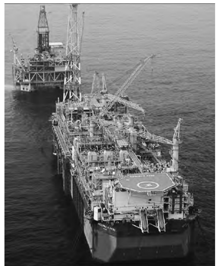
Offshore: Floating oil production, storage and offloading platforms EMBASSY OF THE REPUBLIC OF ANGOLA
