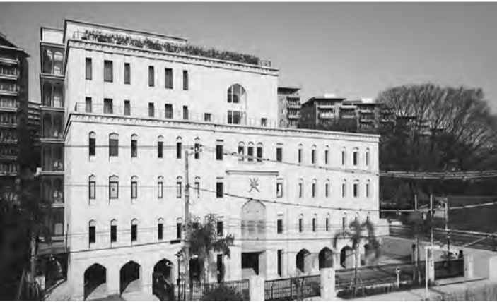
New home: The new building of the Sultanate of Oman's embassy in Tokyo, which is located in Hiroo in Shibuya Ward and opened July 2, 2009. EMBASSY OF THE SULTANATE OF OMAN
