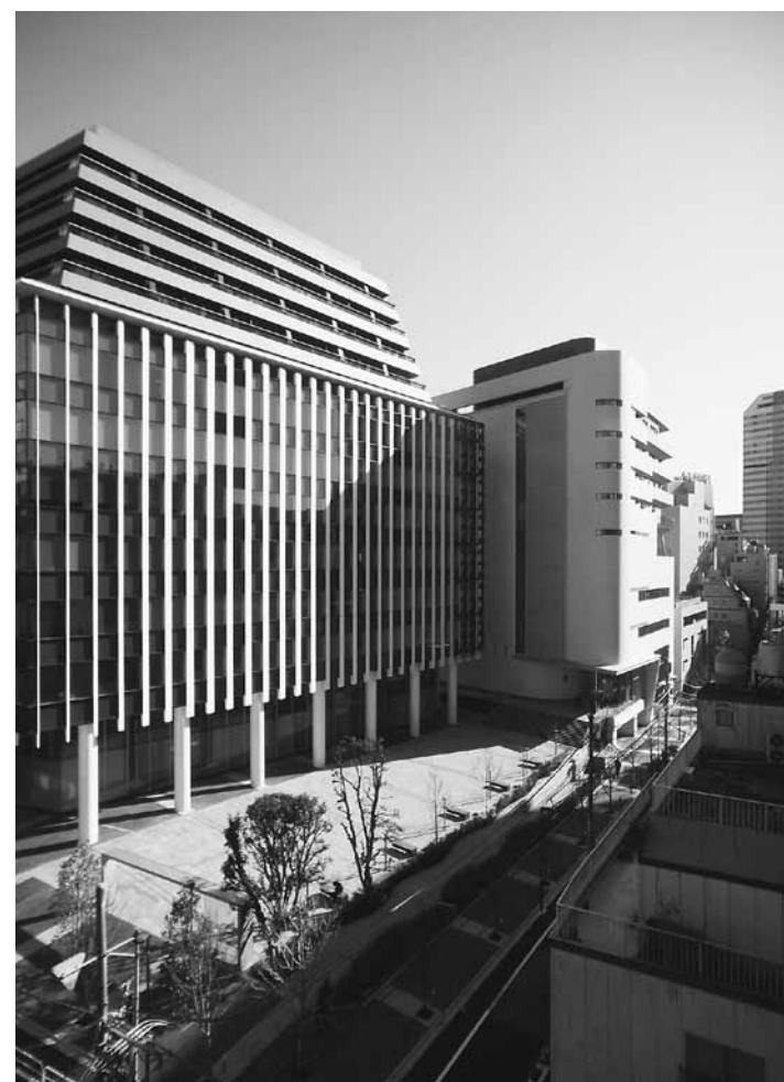
New face: The Belgian Embassy building incorporates limestone from Portugal in its northwest facade. ©NOAN
