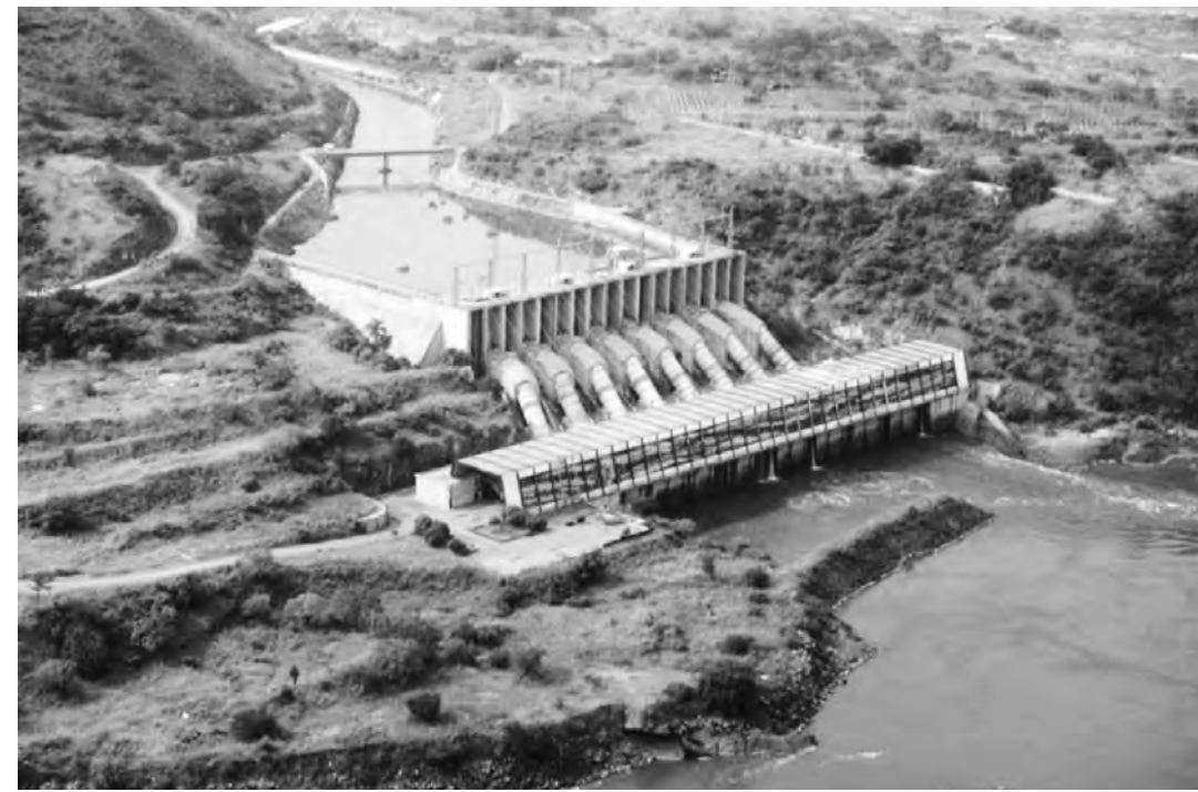
Power spot: Located on the Congo River in Inga, 225 km southwest of the capital Kinshasa, the Inga Dams provide hydroelectricity to the DRC. The smallest, Inga I, was built in 1972, followed by Inga II in 1982. Both are under reconstruction from the damage sustained during the Congo Civil War. Plans for two larger dams, Inga III and Grand Inga, to supply electricity to African countries are in development.
