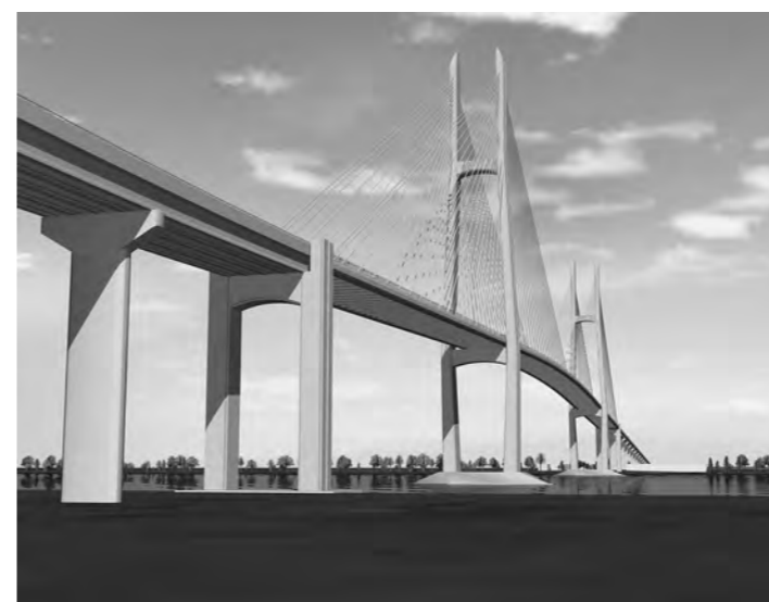
Infrastructure: The longest bridge across the Mekong River will be completed in 2015 with Japan's grant aid.
