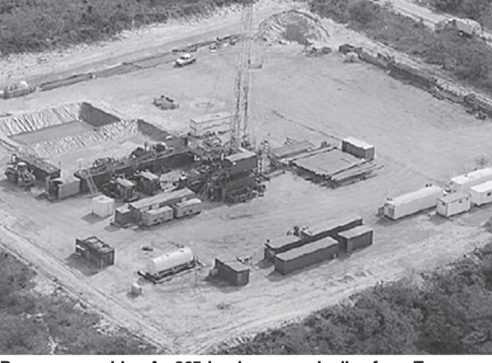
Resource provider: An 865-km-long gas pipeline from Temane and Pande fields (above) supplies gas from Mozambique to South Africa. EMBASSY OF MOZAMBIQUE
