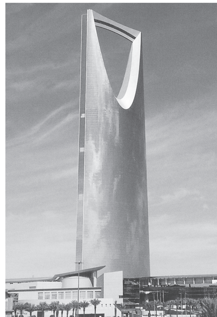
Skyscraper: The Kingdom Centre is a Riyadh landmark and one of the tallest buildings in the Middle East. EMBASSY OF SAUDI ARABIA
