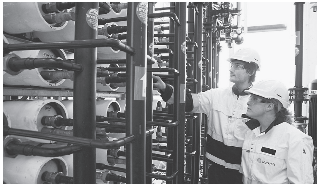
Green technologies: (Clockwise from above) The membranes used for osmotic pressure power generation are coiled up inside pressure vessels; the Middelgrunden wind turbines near Copenhagen, Denmark; the Hellisheidi Geothermal Plant at Mount Hengill, an active volcanic ridge in Iceland. STATKRAFT/EMBASSY OF DENMARK/NATIONAL ENERGY AUTHORITY OF ICELAND
