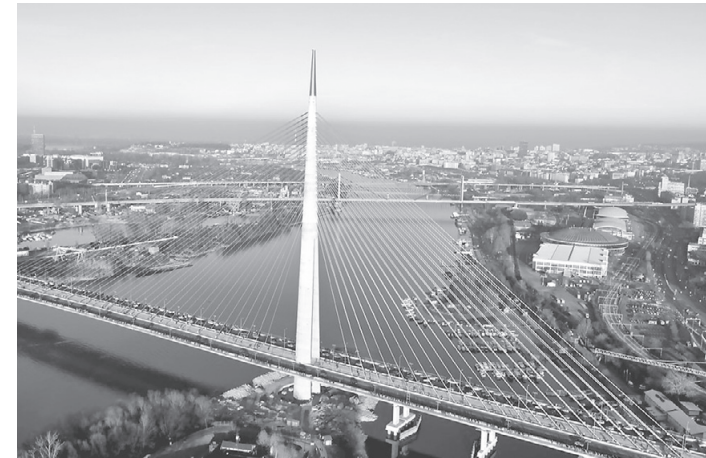
Engineering marvel: Opened this year on Jan. 1, the Ada Bridge spans the River Sava and connects Cukarica and New Belgrade, two of the capital's municipalities. EMBASSY OF SERBIA
