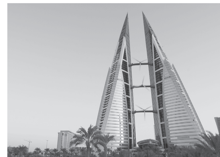
Futuristic: Built in 2008, the Bahrain World Trade Center is the first skyscraper in the world to integrate wind turbines into its design. EMBASSY OF BAHRAIN
