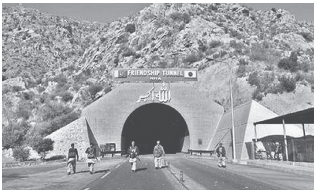
Cooperation: Constructed with Japanese assistance, the 1.9-km long Kohat Tunnel, also known as the Pak-Japan Friendship Tunnel, serves as a shorter, alternate route to the Kohat Pass in the northwest frontier of the country. EMBASSY OF PAKISTAN
