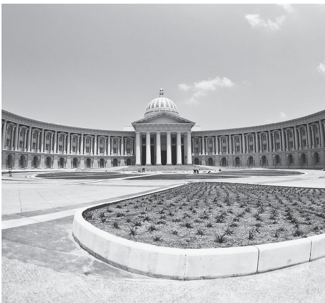
Classical modernity: Inaugurated in 2009, the second unit of the Global Education Center on the Infosys campus in Mysore, India, is where all Infosys employees undergo training before their placements. The GEC is the largest corporate education center in the world. EMBASSY OF INDIA
