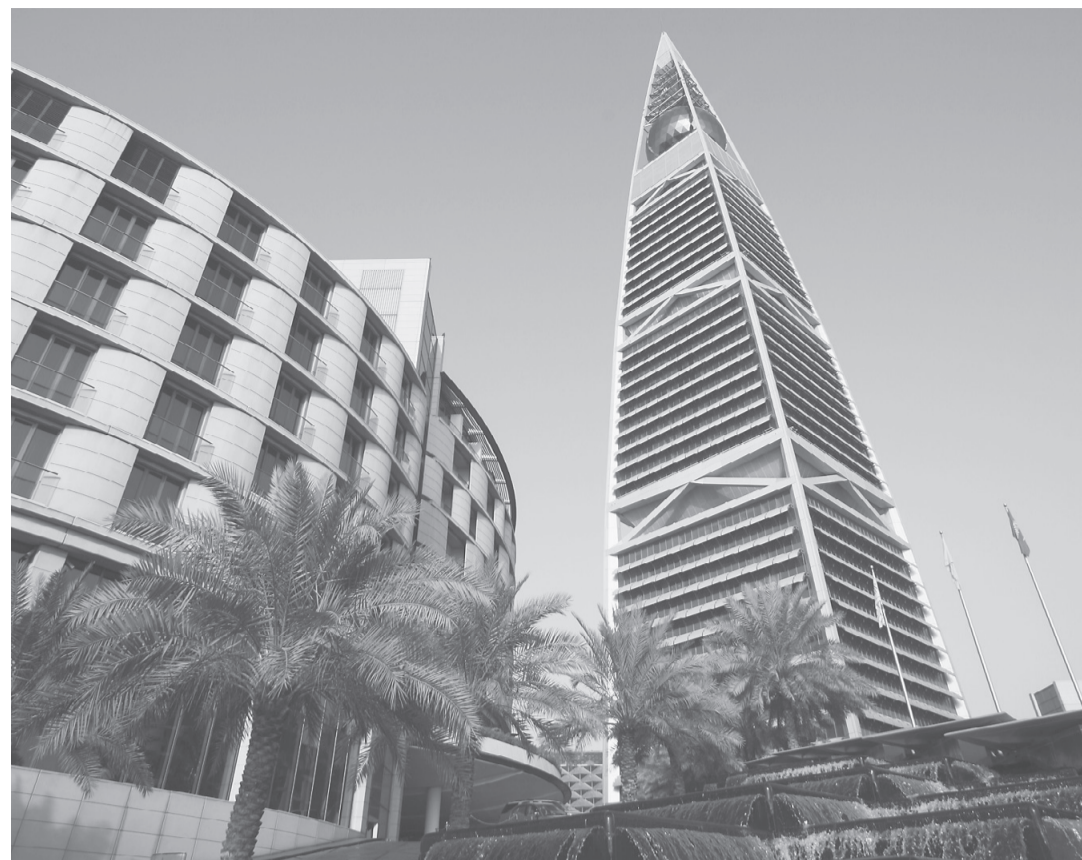
Riyadh icon: Al Faisaliah Tower was the first of the startling new structures to rise above the Saudi Arabian capital's skyline. On its 34 floors there is a five-star hotel, four exclusive restaurants, a shopping mall, offices and apartments. The needlepoint pinnacle is 267 meters above the ground. EMBASSY OF SAUDI ARABIA
