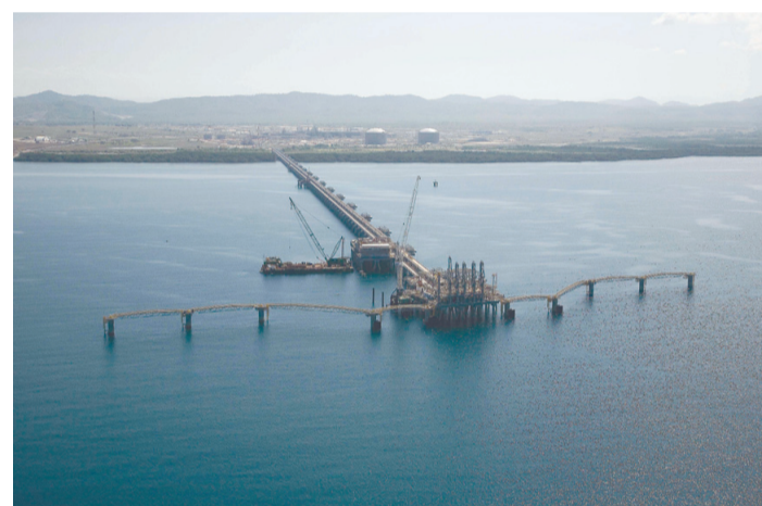
Natural resources: The construction phase of Papua New Guinea's first liquefied natural gas project will be completed by the end of this year. EMBASSY OF PAPUA NEW GUINEA
