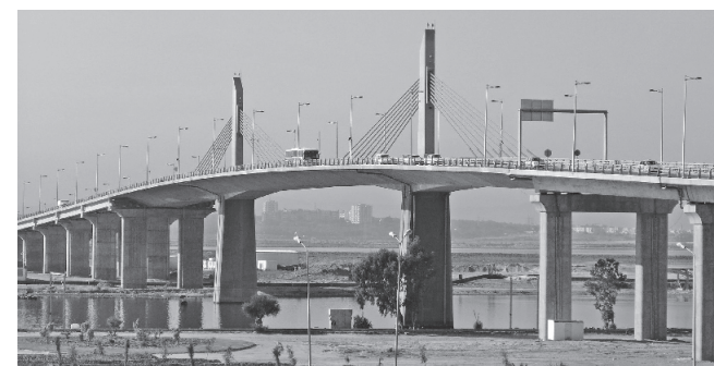
With pride, TAISEI CORP. accomplished La Goulette Bridge, opened on March 21, 2009.
