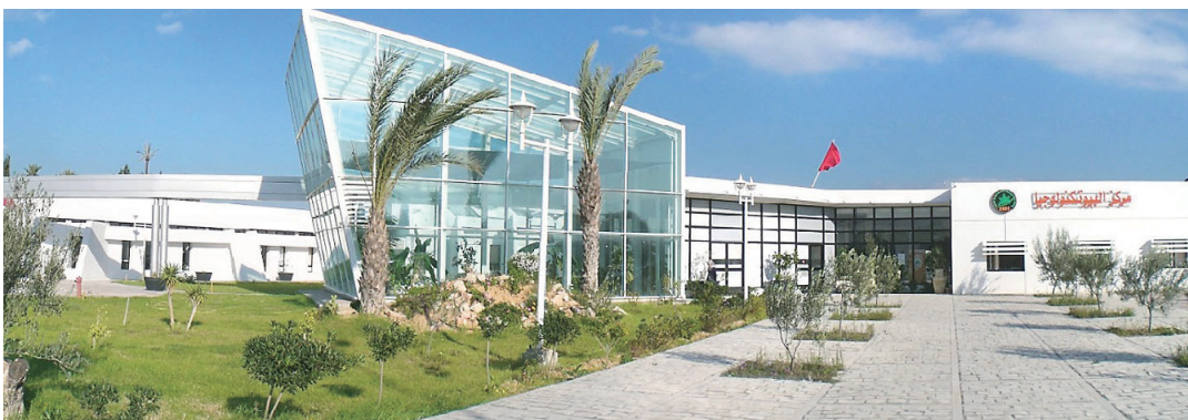
Borj Cedria Technopark is an example of Tunisian-Japanese cooperation. EMBASSY OF TUNISIA
