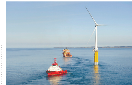
The Hywind floating wind turbine being deployed in the North Sea.
