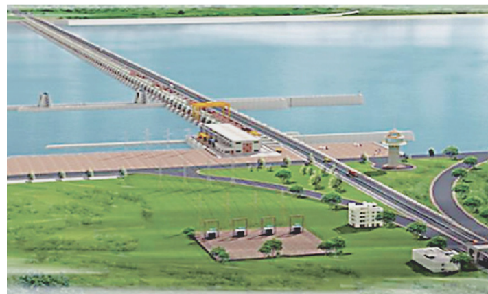
Padma Bridge, which is currently under construction EMBASSY OF BANGLADESH
