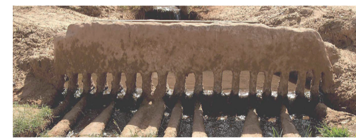
Foggara, a traditional system for agriculture irrigation, was studied by the late professor Iwao Kobori. EMBASSY OF ALGERIA
