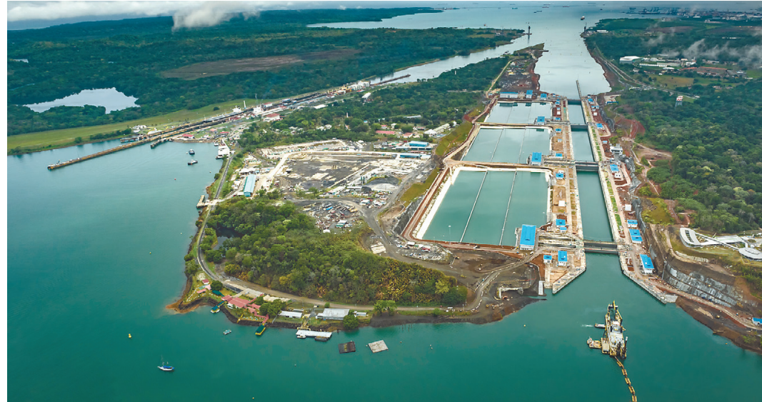
Panama Canal expansion PANAMA CANAL AUTHORITY
