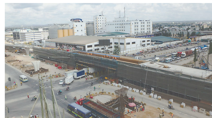
Top: Zanzibar Island in the Indian Ocean is one of the most popular tourist sites in Tanzania. Above: The Tazara flyover is being constructed by Sumitomo Mitsui Construction Co. at a critical junction of roads leading to the port and airport in Dar es Salaam.
