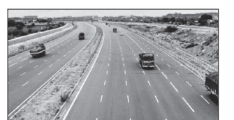
CPEC ROAD PROJECT
