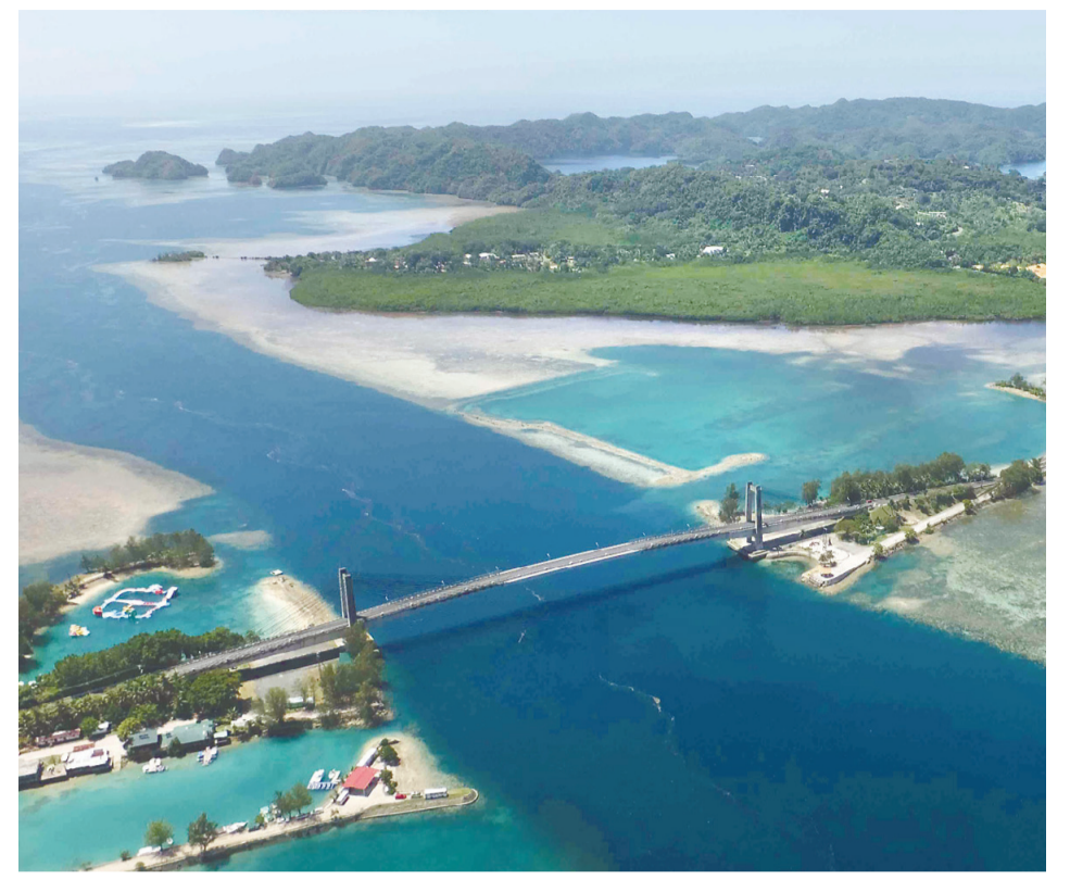
The Japan-Palau Friendship Bridge acts as the main artery of the country. The bridge connects Palau's two major islands: Koror and Babeldaob. EMBASSY OF THE REPUBLIC OF PALAU
