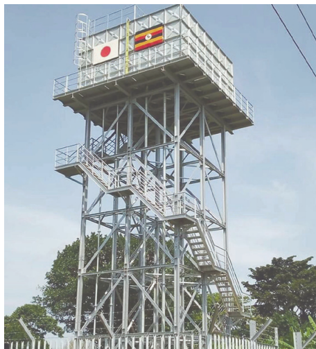
Japan continues to support water supply systems in Uganda. EMBASSY OF JAPAN IN UGANDA / JICA
