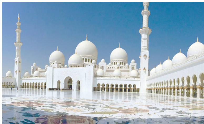
Sheikh Zayed Grand Mosque EMBASSY OF THE UAE
