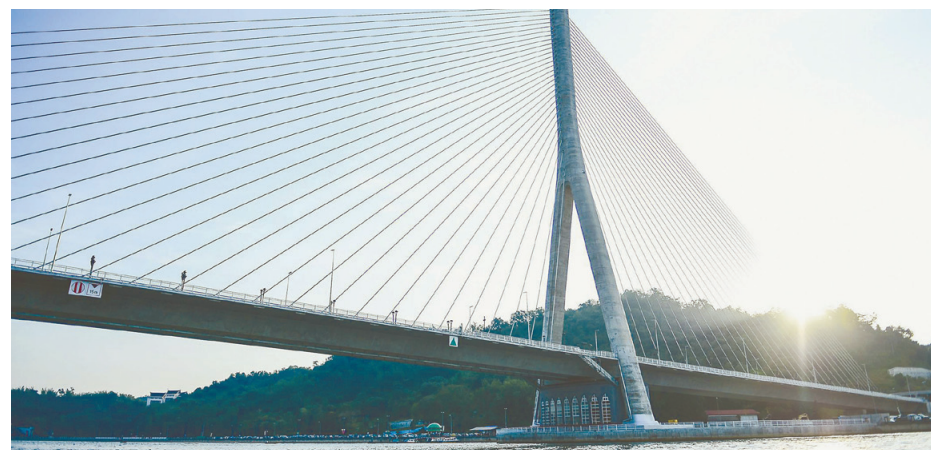
The Raja Isteri Pengiran Anak Hajah Saleha Bridge, commonly known as the Sungai Kebun Bridge, opened in October 2017. The bridge connects Kampung Sungai Kebun to Bandar Seri Begawan.
