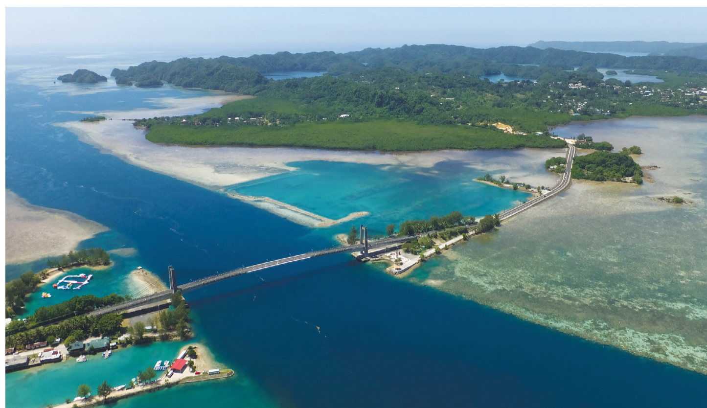
The Japan-Palau Friendship Bridge, built with Japan's official development assistance and completed in 2002, connects the islands of Koror and Babeldaob. NARIHIRO TANAKA
