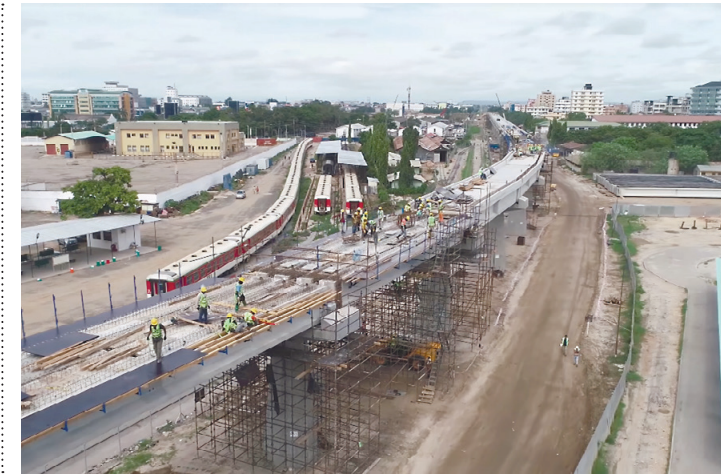
The section of the Tanzania Standard Gauge Railway between Dar es Salaam and Morogoro, currently under construction
